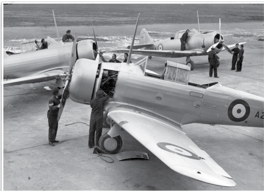
RAAF maintenance personnel inspecting three Australian made CAC Wirraway aircraft
