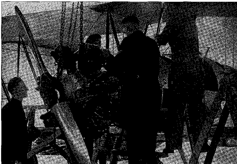
Figure 1.2 Mechanics installing an engine in an Avro Trainer. 19
